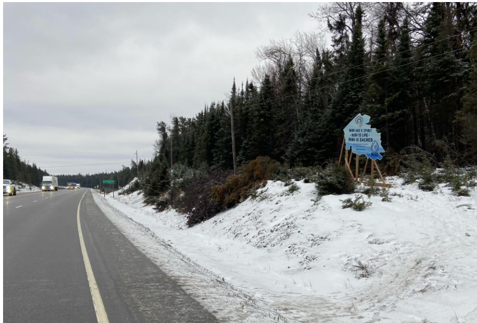
Photo of the western nibi sign after installation.
